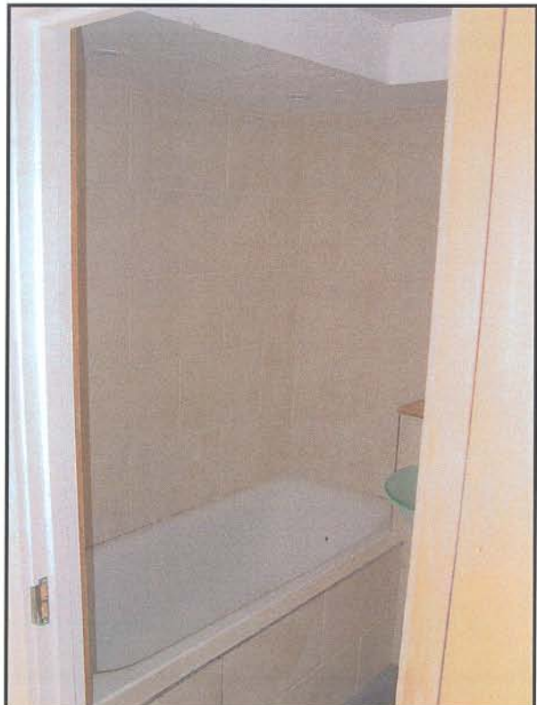
BATHROOM FLAT 13 (5 TH FLOOR)
